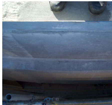
Figure 10. Feathered edge box out after repair.
