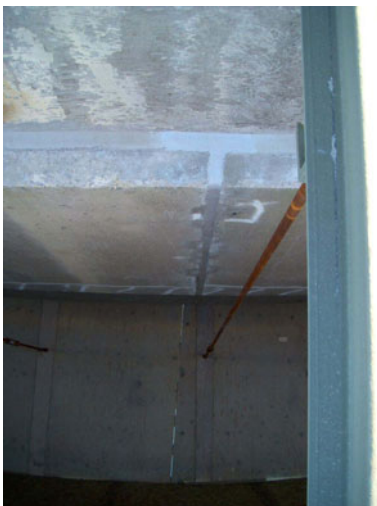
Figure 7. Repaired joint sealant (horizontal and vertical) of the concrete overlay.
