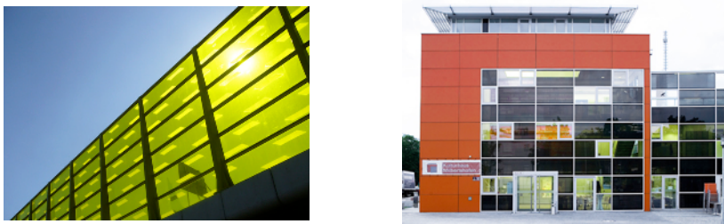
Fig. 2. (left) Example of potential application as soundbarrier; (right) example of potential application in the building envelope.
