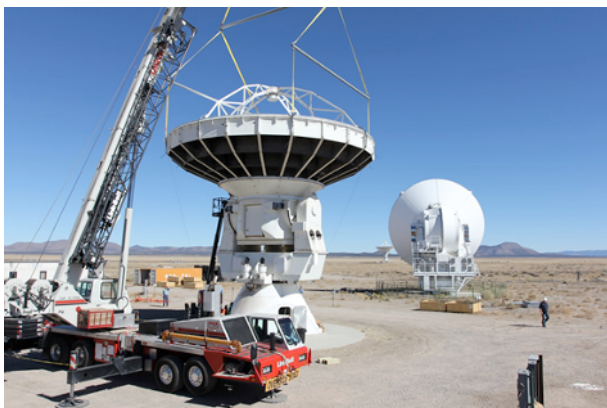
Figure 5. Disassemble one of the ALMA prototype antennas for retrofitting and ready to operate in the extremely cold environment on the Greenland ice sheet. This picture shows the disassembly process in November 2012, at the site of the Very Large Array near Socorro, New Mexico. This effort is led by ASIAA personnel, Philippe Raffin, Ted Huang, and George Nystrom, in collaboration with the engineers from Aeronautical Research Laboratory.
