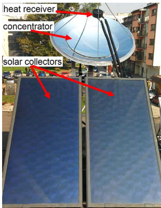
Fig. 1 View of the hybrid system of solar panels and solar radiation concentrator mounted on the roof of Department of Sustainable Energy Development, AGH University in Krakow.
