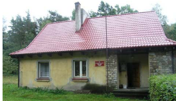
Fig. 1. A view of the western façade of Forest Lodge 2 after partial thermal upgrading (roof replacement), the photograph by Piotr Szafraniec, Świętokrzyski National Park.
