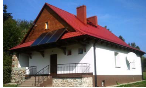
Fig. 3. A view of the eastern and southern façades of Forest Lodge 2 after thermal upgrading (solar collectors installed), the photograph by Piotr Szafraniec, Świętokrzyski National Park.
