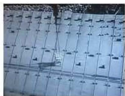
⑳ Iron shield* plates on the DS pool *15cm thick
