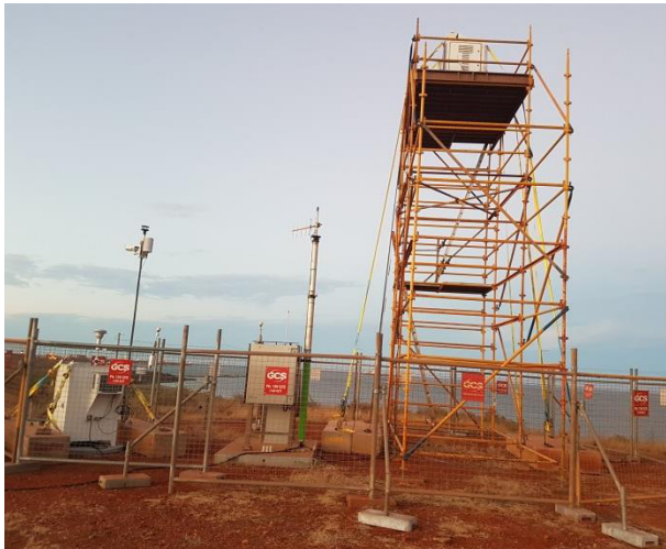
Figure 2 WINDCUBE200S and BAMS installation on site 1
