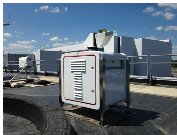
Figure 2 – Installations of WINDCUBE100S lidar and MP3000a radiometer at University of Albany
