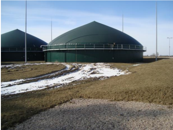
Fig. 1. View of fermentation chambers in the Ryboly biogas plant.
