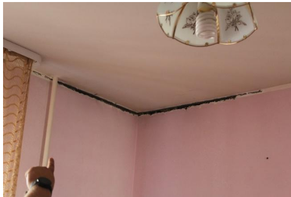
Fig. 4. Examples of cracks that formed between floor slabs and vertical wall filling.
