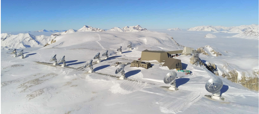
Figure 1. View of the NOEMA observatory as seen from the southeast. The antennas are arranged in the most compact configuration. The observatory is located in the French Alps at an altitude of 2550 m above sea level. NOEMA is operated by IRAM, an international research institute supported by the CNRS (France), MPG (Germany) and IGN (Spain). Photo by J. Boissier.
