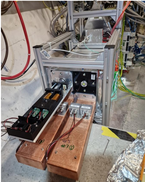
Fig. 8. Upgraded PMT system during installation.
