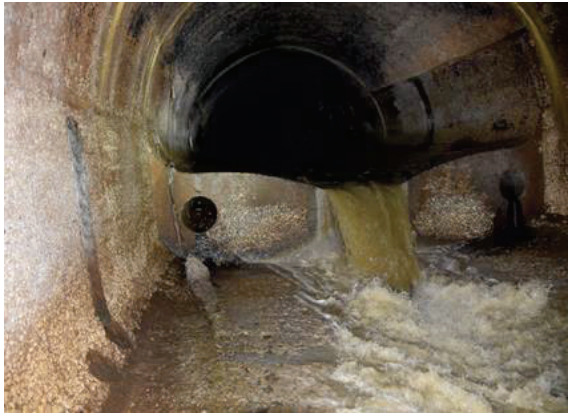
Fig. 5. Alcântara large sewer collector in the underground region of Campolide.
