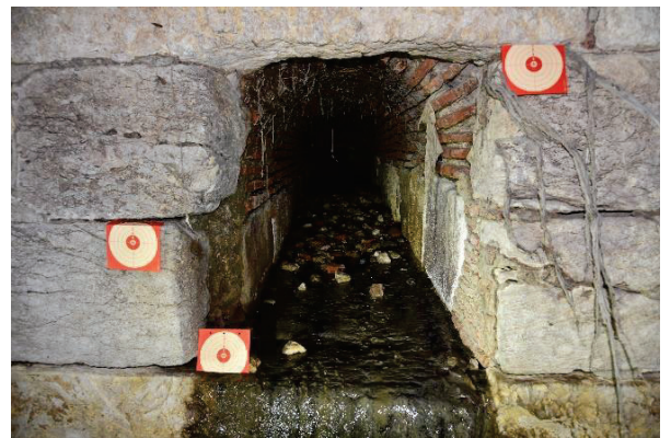
Fig. 3. Image of the digitalized region in the sewer.
