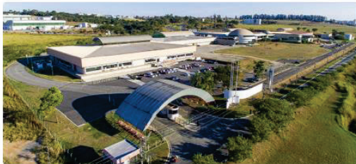
Fig. 1. Panoramic view of the Technological Innovation Park (PIT)
