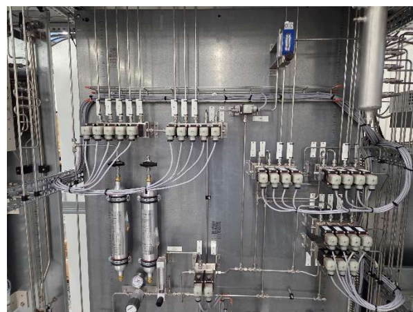
Fig. 3. Secondary sampling system in green H 2 production
