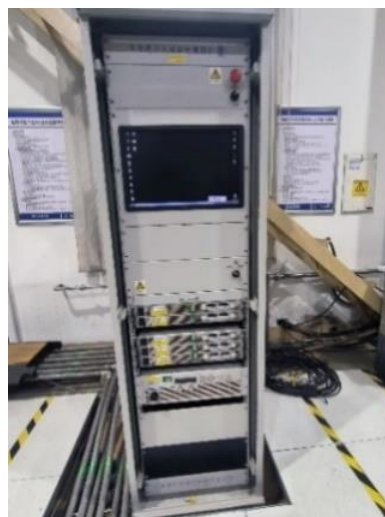
Fig. 5 Power source for hall thruster testing
