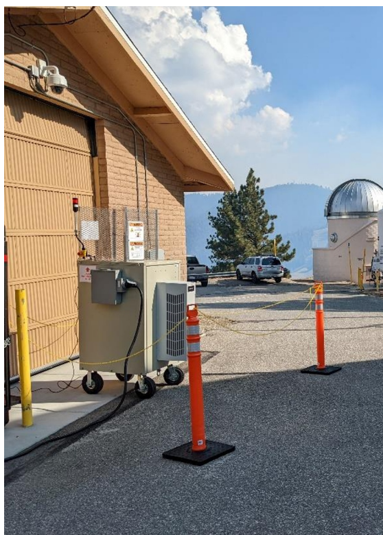
Figure 1. The SMOL system at JPL Table Mountain Facility.
