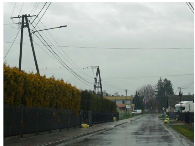
Fig. 1. Example of installing street lighting luminaires on power line poles.
